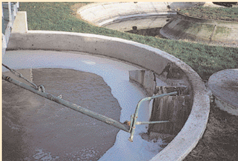
Station d'épuration, désablement ▶
